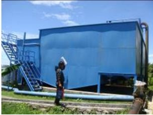
Picture 3.5 WTP Nemewikarya paket steel capacity 40 l/sec
