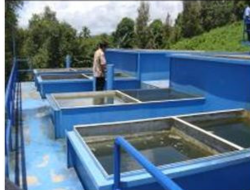
Picture 3.5 WTP Nemewikarya paket steel capacity 40 l/sec
