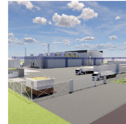
Waterstoffabriek VoltH2 & Virya Energy in North Sea Port
