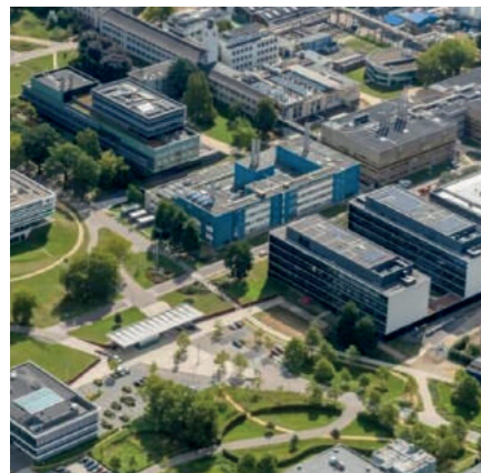
Proeffabriek Deep Branch op Chemelot in Limburg
